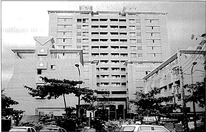
Living quality of servicemen and their dependents improved substantially through the rebuilding of military dependent quarters.
