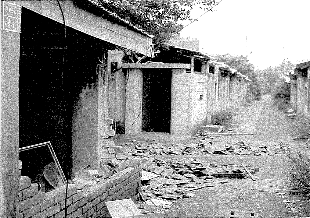
Original appearance of Chang Feng 3rd Quarter before rebuilding
